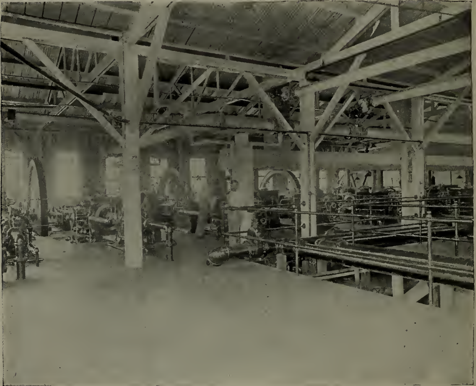
Interior of Weehawken Air Compressor Plant for P.R.R. North River Tunnels.
